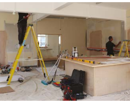
Pictured: The build process Photo credit: Milton Abbey School
